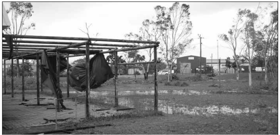
Cyclone damage at the Mt Louisa House of Praise youth centre
